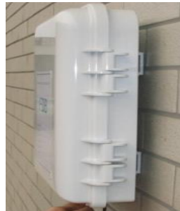
FDB fiber termination box on the wall
