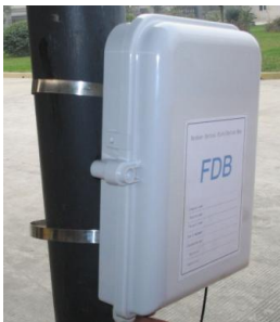
FDB fiber termination box on the pole
