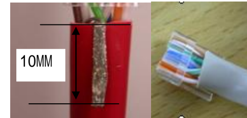
6. Cut the Balance Wires
